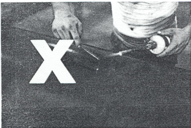
3. Melt the "E-Z Stick" onto the surface.
